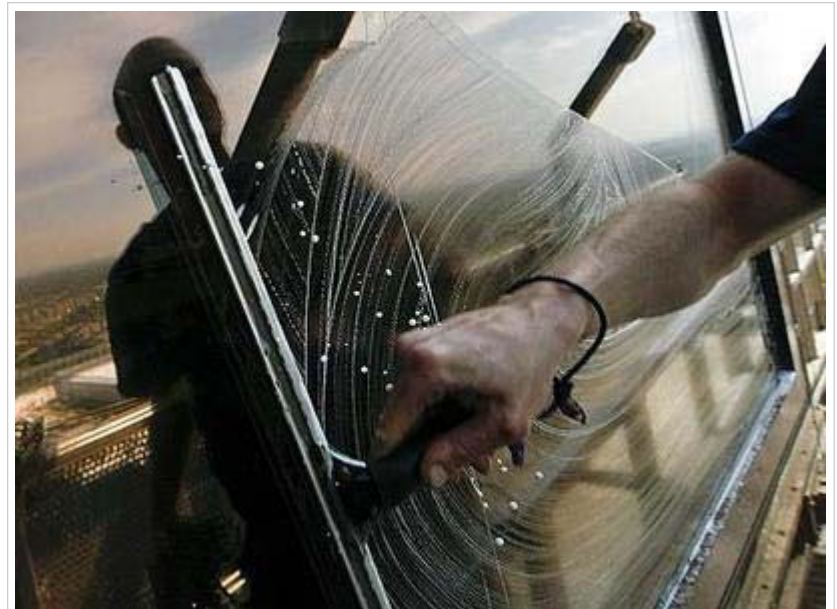
Trevor Pitts, who has wielded a squeegee for three years, wipes a window high up the 70-storey Scotia Plaza building, which can take 10 weeks to clean.
